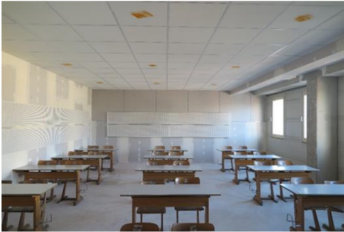
Figure 3: Classroom with acoustical suspended ceiling and classroom furnishing. Additionally shown are sound absorbers on the walls, which are installed in the middle of the wall surface at ear level of seated persons.
